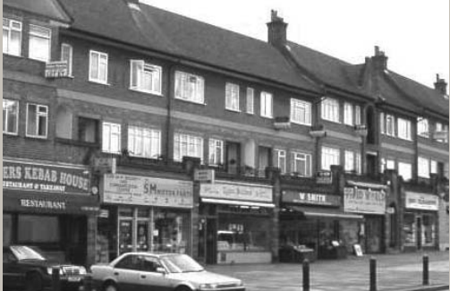
Simple traditional shopfront with narrow fascia
